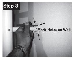
Slide Wall Mount Flanges (#6) into Wall Mount Tubes (#7) Place unit against wall where it is to be mounted and mark Wall Flange holes.
