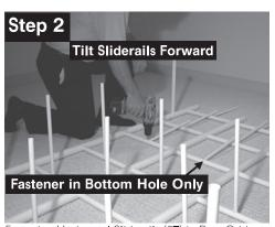
Fastening Horizontal Sliderails (**#7**) in Rear Grid using 18 - #06 x 1/2" Fastening Screws (**#1**) *Tip: Start at top row and work down*
