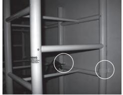
Note: If mounting into Drywall or Masonry, mark & drill 1/4" holes and insert plastic wall anchors - and proceed with step 1-
