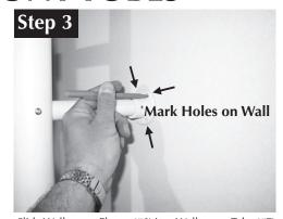
Slide Wallmount Flange (#6) into Wallmount Tube (#7) Place unit against wall where it is to be mounted and mark Wall Flange holes.
