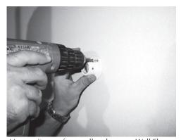
Move unit away from wall and remove Wall Flange from Tube and mount Flange to wall using 12 #10 x 1-1/4" Wall Mount Flange Screws (#3) and Plastic Wall Anchors (#4) if needed.
