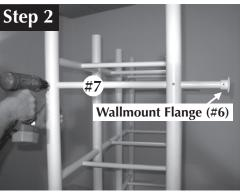
Move unit away from wall and insert 4 Wallmount Extension Tubes (#7) at 4 Locations. Fasten With 8 - #08 x 3/4" Extension Tube Fastening Screws (#2) Note: 1 Fastener Per Joint Front Side Only
