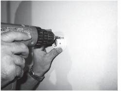
Move unit away from wall and remove Wall Flanges from Tubes and mount Flanges to wall using 12 #10 x 1-1/2" Wall Mount Flange Screws (#3) and Plastic Wall Anchors (#4) if needed.
