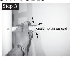
Slide Wallmount Flange (#6) into Wallmount Tube (#7) Place unit against wall where it is to be mounted and mark Wall Flange holes.
