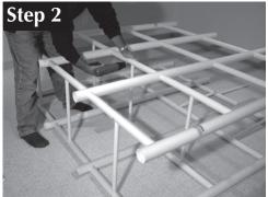
Insert and fasten next 3 rows of Sliderail to Front Grid using 9 - #06 x 1/2" Fastening Screws (#1) Note: Fasteners in Bottom Hole Only
